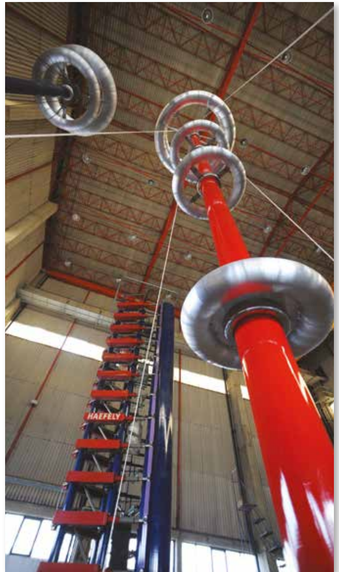
Lightning impulse generator voltage divider.
