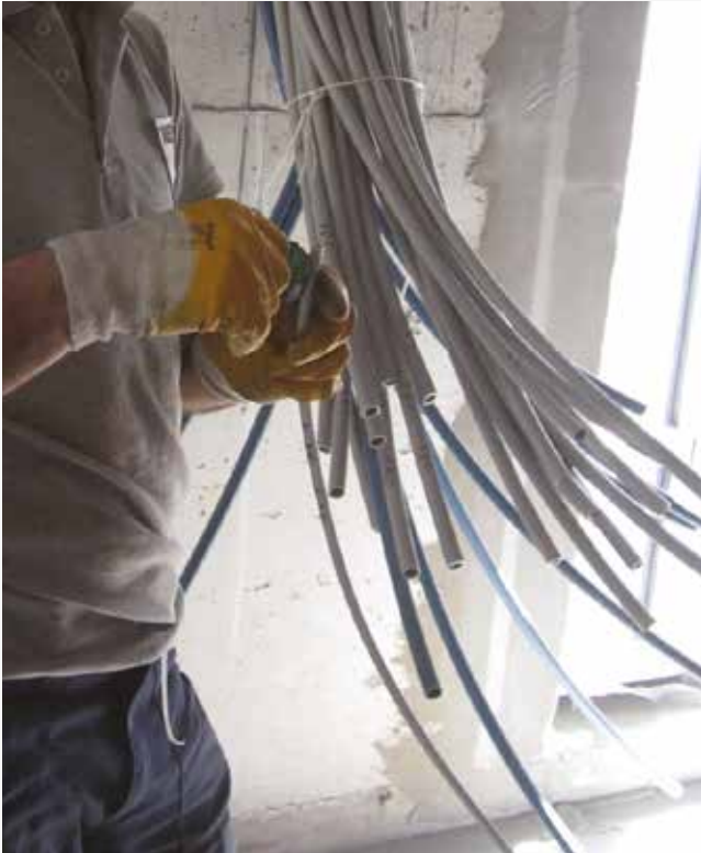
An operator stripping cables during installation.
